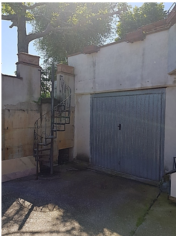
Figura 15 Accesso al locale garage_Fg. 2 part 1472 sub 2
