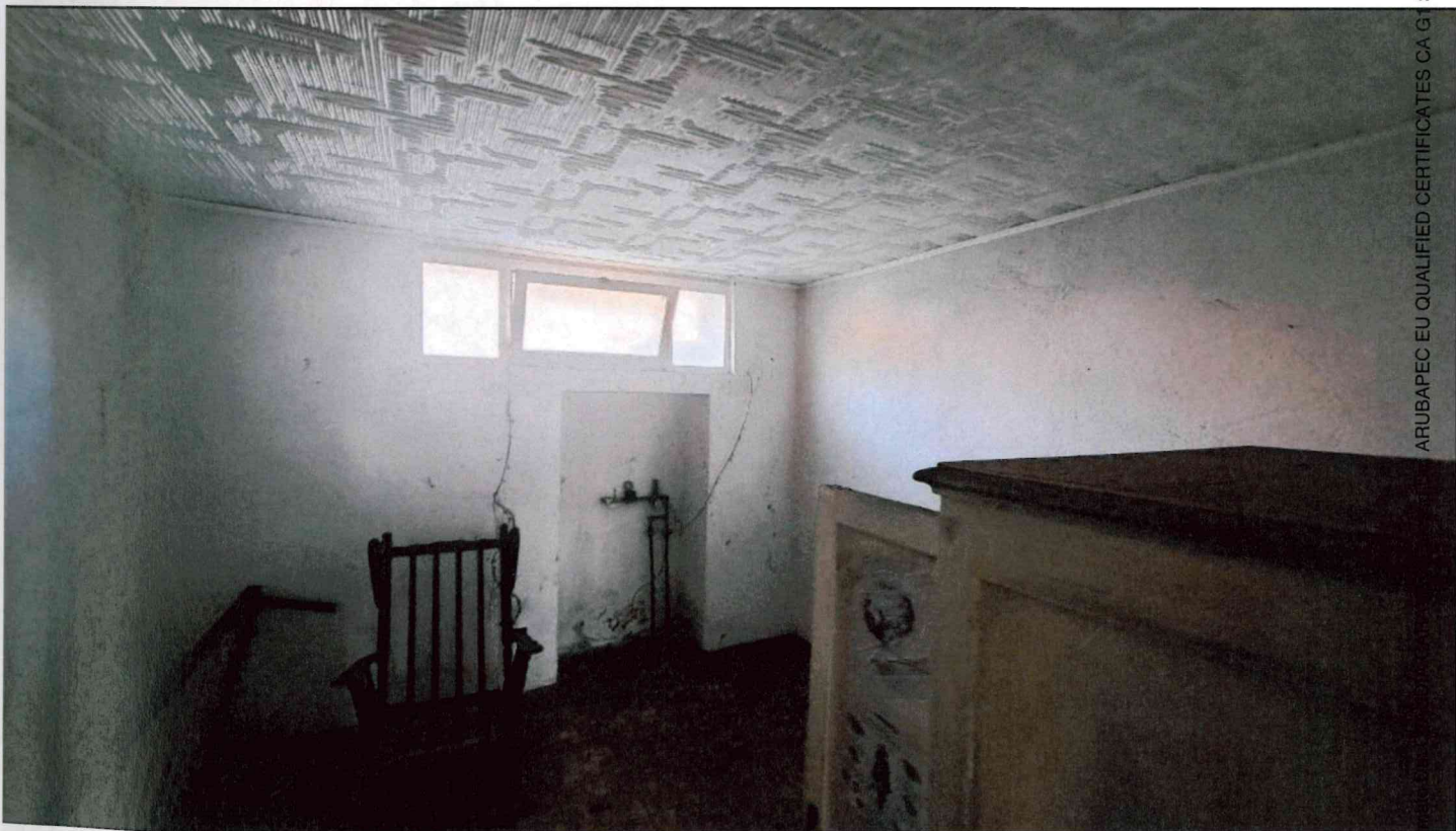
Piano seminterrato cantina
