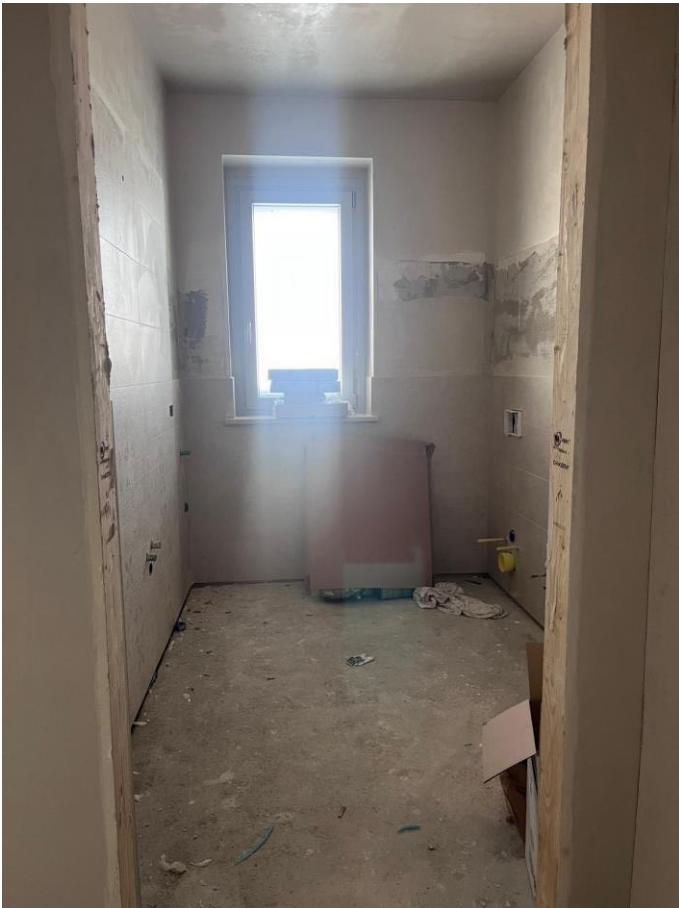
piano terra – bagno
