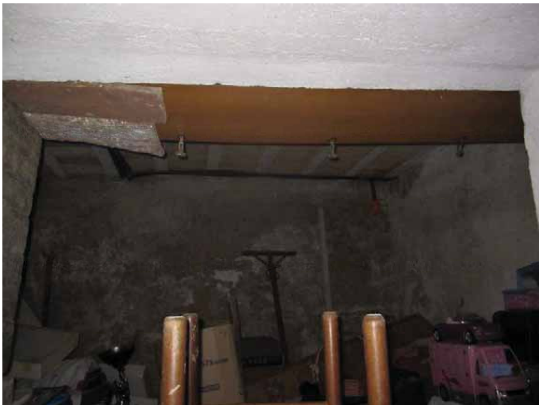
PIANO TERRA CANTINA
