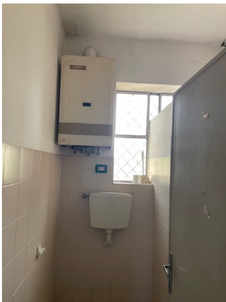
Bagno – wc piano terra
