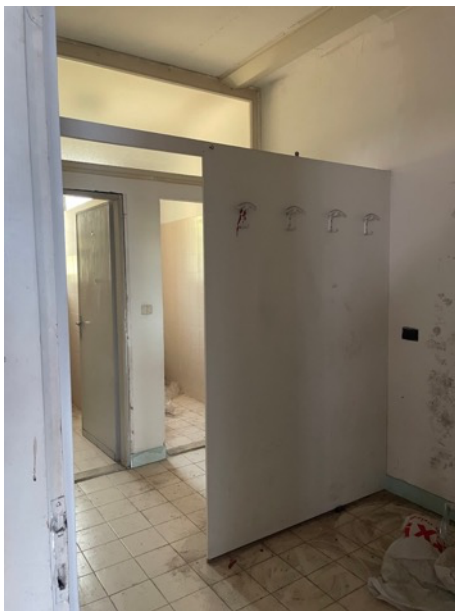
Antibagno piano terra
