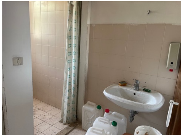
Antibagno piano terra
