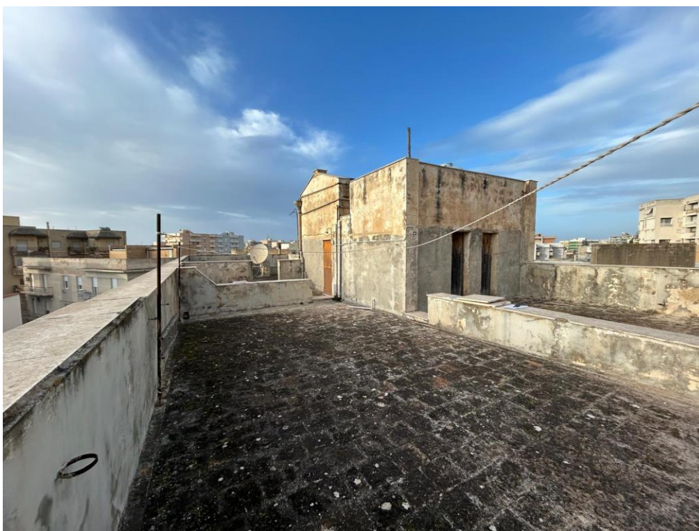
Piano terrazzo – locale lavanderia
